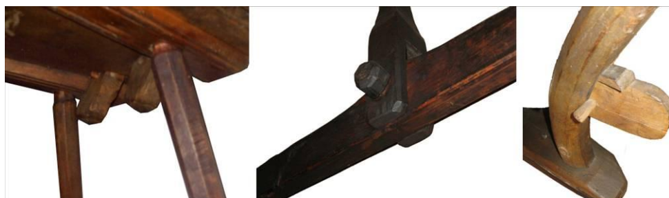
Fig. 6 – Examples of the wooden spigot type joints (The Wood Museum in Campulung Moldovenesc, Suceava, Village Museum, Suceava; Ethnographic Parc "Romulus Vuia", Cluj Napoca) (Photo designer Ilarion Constantin Balan)
