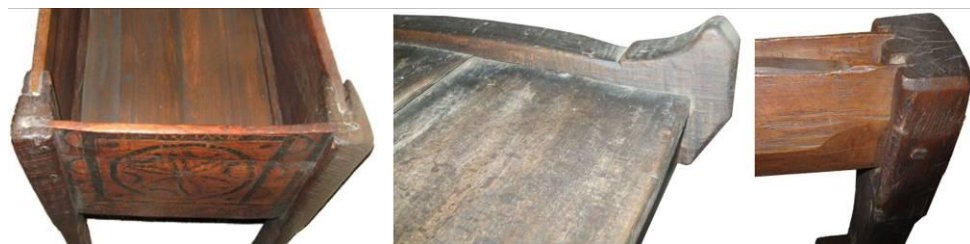
Fig. 10 – Examples of overlapped spigot joints (The Wood Museum in Campulung Moldovenesc, Suceava; Ethnographic Parc "Romulus Vuia", Cluj Napoca) (Photo designer Ilarion Constantin Balan)
